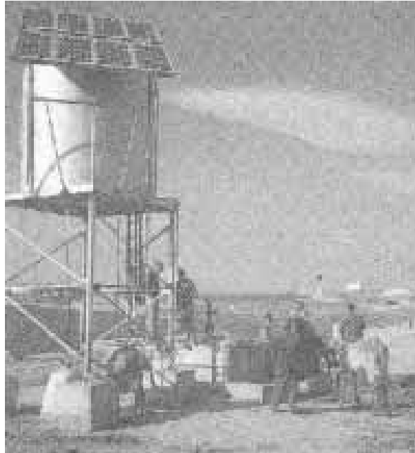
Figure 5: Photovoltaic pumping system in Tunisia
