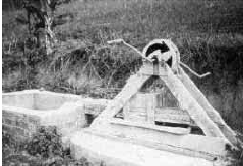
Figure 1: Hand-operated reciprocal pumping system
