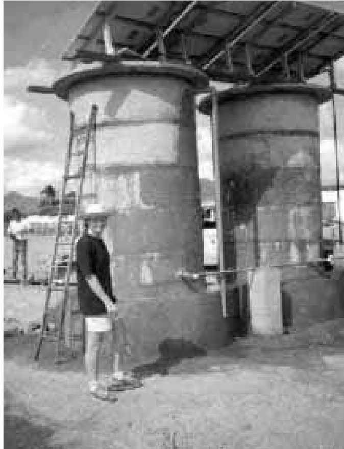
Figure 52: PVPS with water tanks in Brazil
