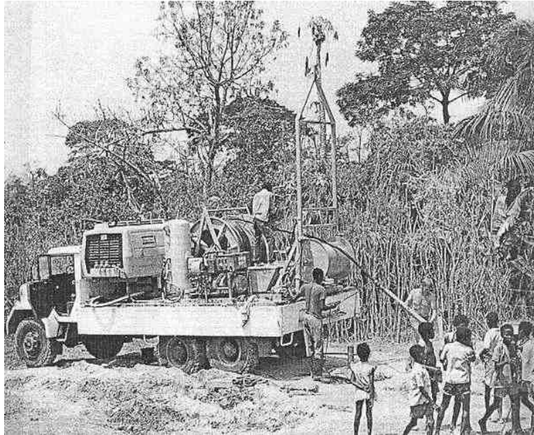
Figure 38: Installation of a pump in a well in Ghana (/16/ Sandomeer, 1985)
