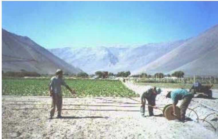
Laying pipes with integrated labyrinth drippers
